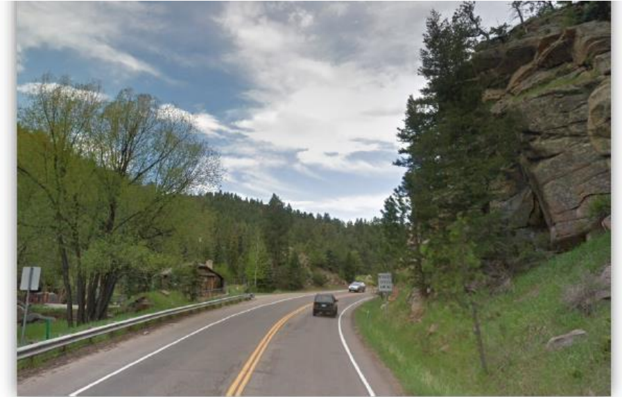
CDOT applied design guidelines and visual mitigation goals to create naturalized rock cuts and to retain native forest vegetation along SH 74 (Evergreen Parkway) using an interdisciplinary design process.
