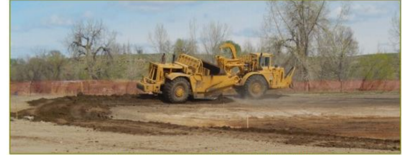
Topsoil placement upon completed cut and fill slopes (207.04)
